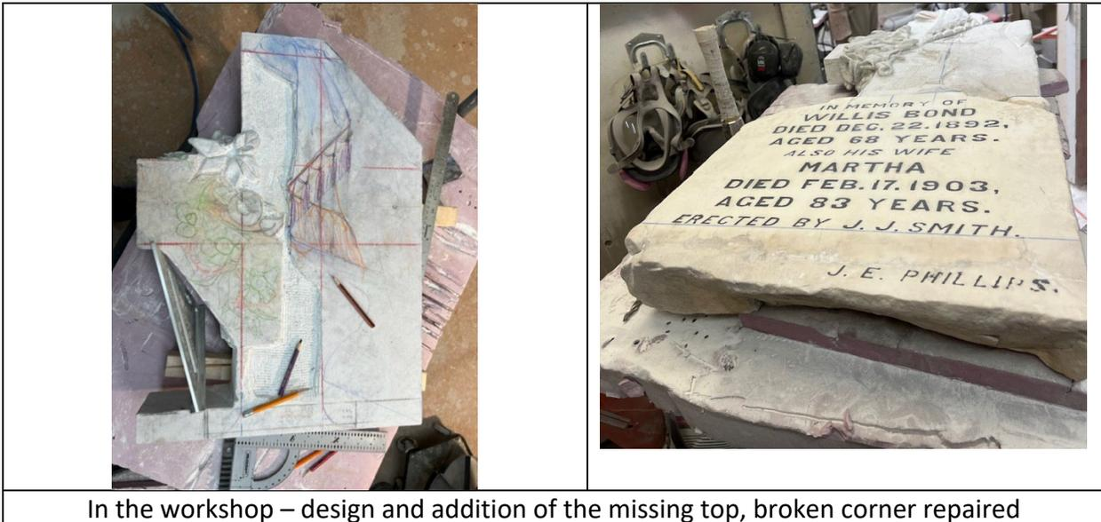
In the workshop – design and addition of the missing top, broken corner repaired
